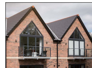
① Ashington Red Multi facing brickwork
