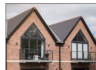
① Ashington Red Multi facing brickwork
